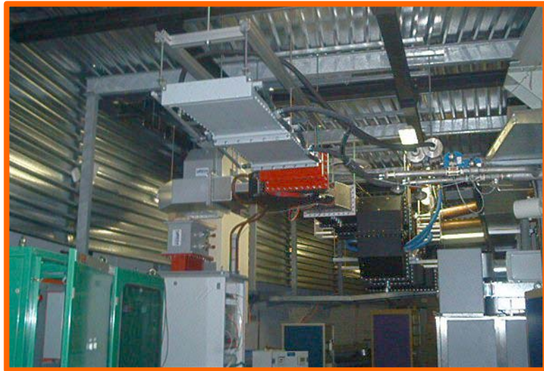
Waveguides for the 150 kW 500 MHz cw plant at elettra
