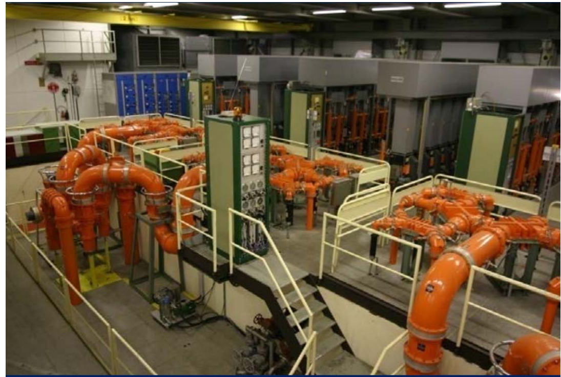
SPS (CERN) Philips 4x550kW 72 tetrode amplifiers
