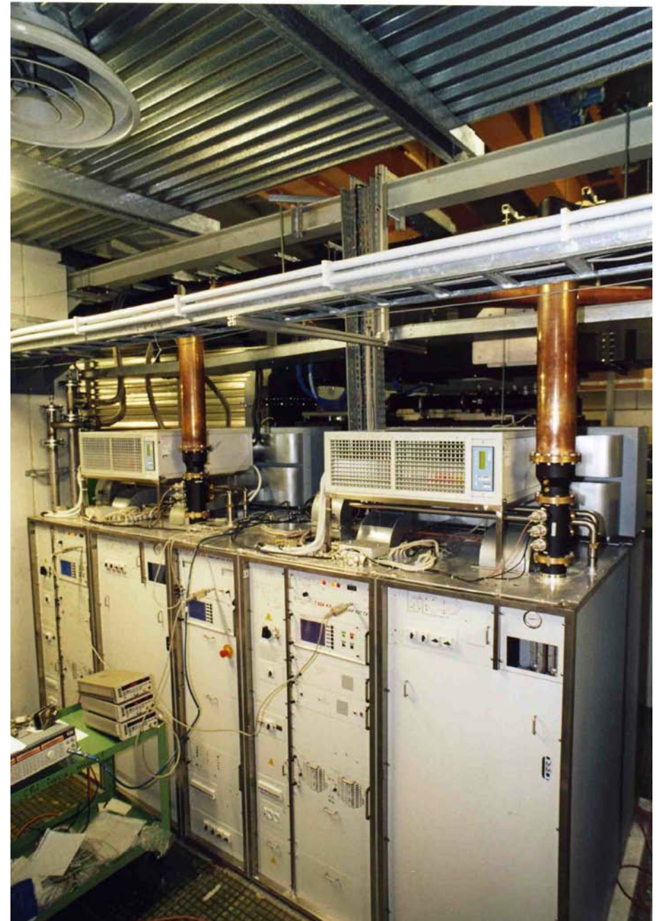
150 kW amplifier combining 2 x 80 kW IOTs in Elettra
