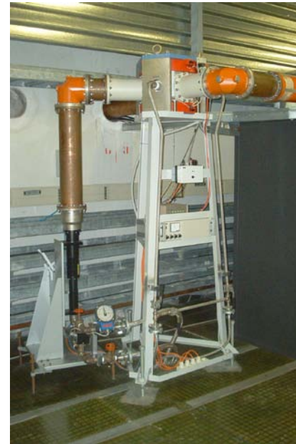
Circulator, load and coaxial lines for the 500 MHz Elettra plants
