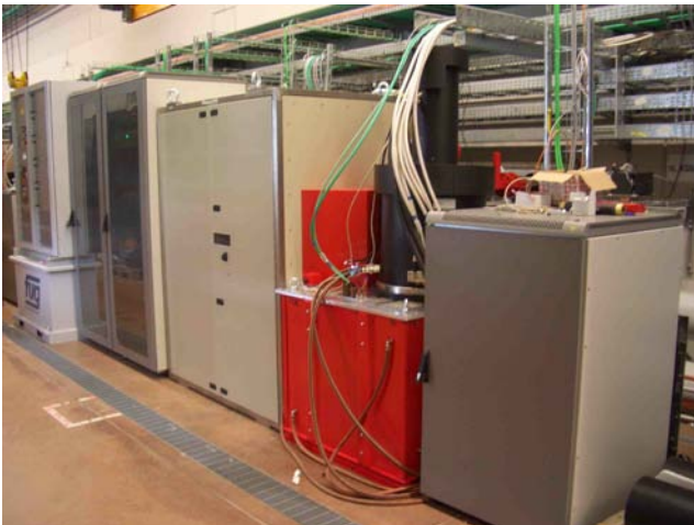
45 MW peak S-band klystron and modulator at FERMI
